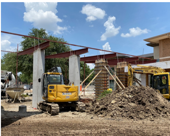
Left - Concrete poured around the Corrigan Porte Cochere area. Right (Top) - Exterior sheathing installed at the Corrigan Auditorium. Left (Bottom) - Roofing in progress in the Corrigan dining areas.
